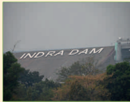
Lower Indra Irrigation Project
