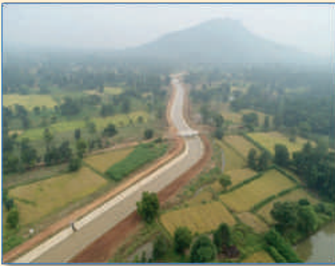
Upper Indravati Lift canal
