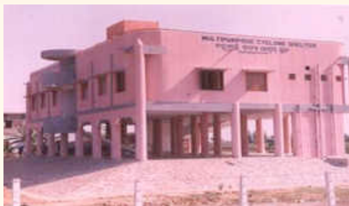
Multipurpose Cyclone Shelter Source: OSDMA
