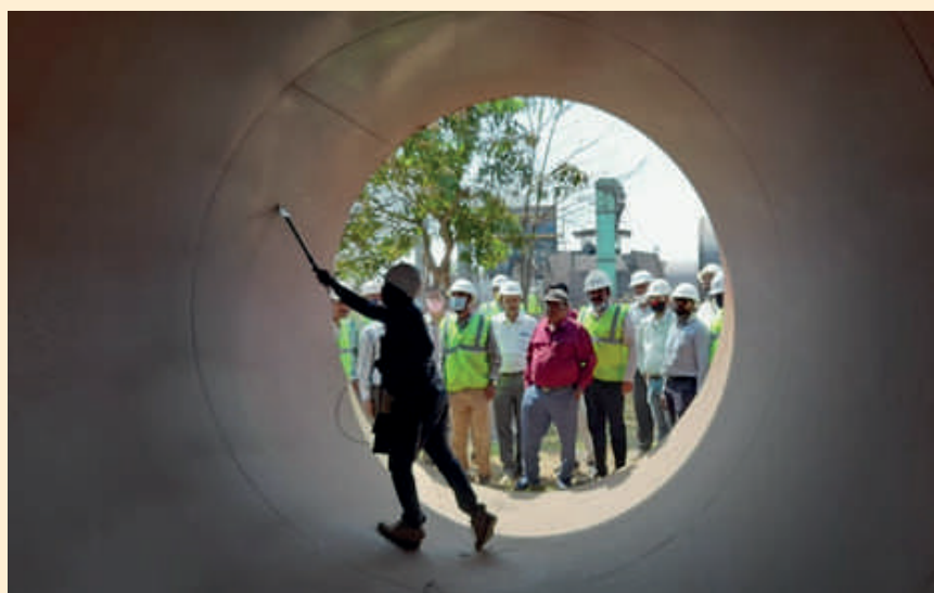
Gangadhar Meher Lift Canal Project (Underground pipeline for Canal Irrigation)
